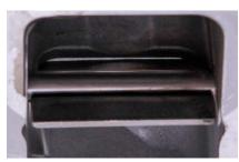
The cooling cannot be regulated if the bypass damper does not close densely.
